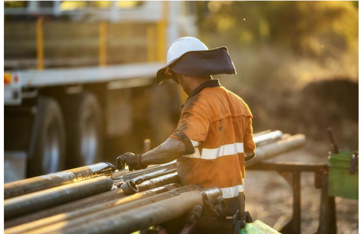
Drill rig in action during the recently completed Phase V drilling program
