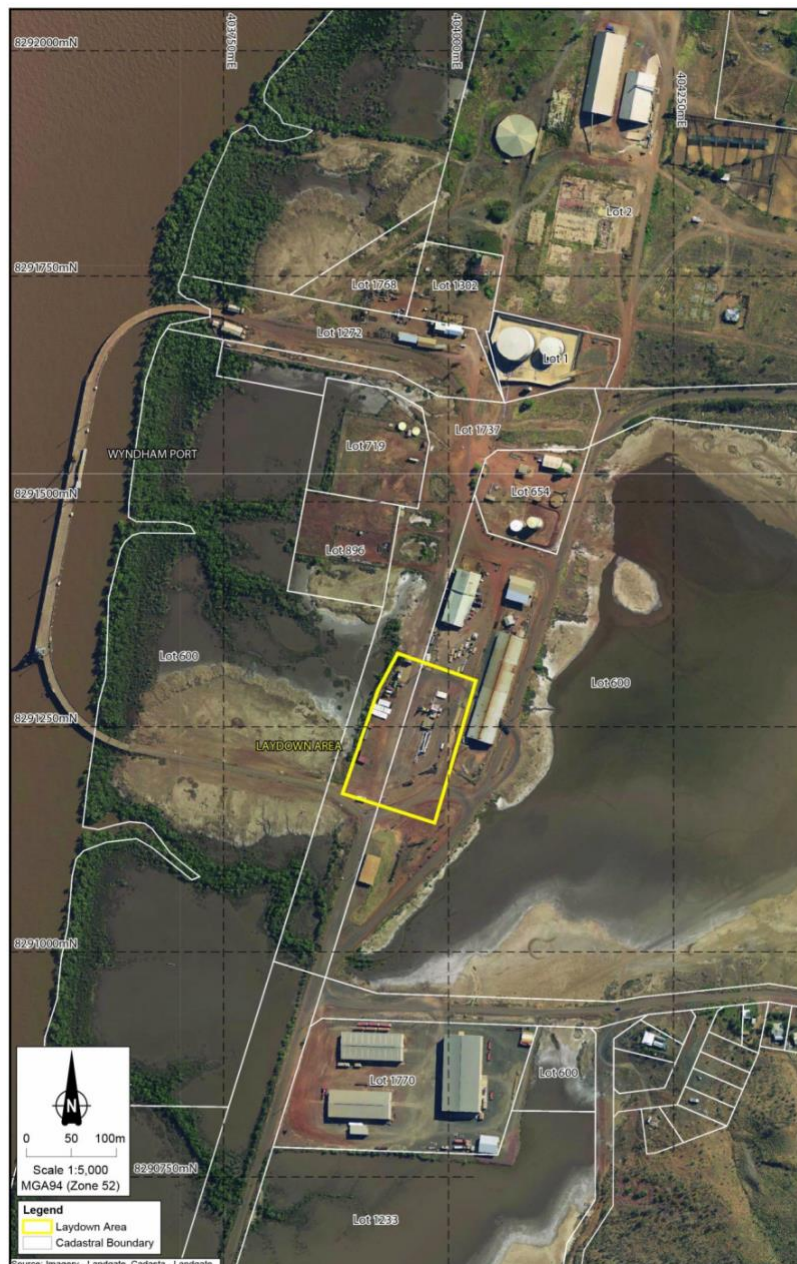
Figure 3 Port of Wyndham and the area set aside for the Sorby Hills port facilities
