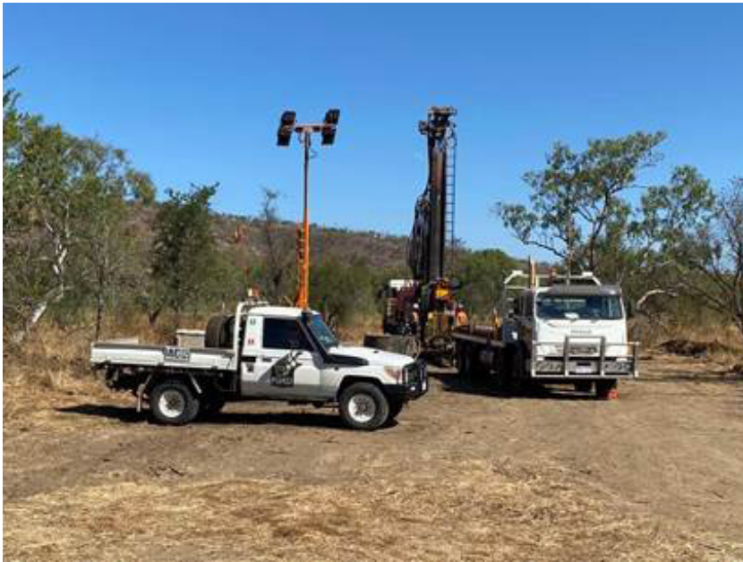
Fig 2. Diamond Drilling at the Wildcat Target
