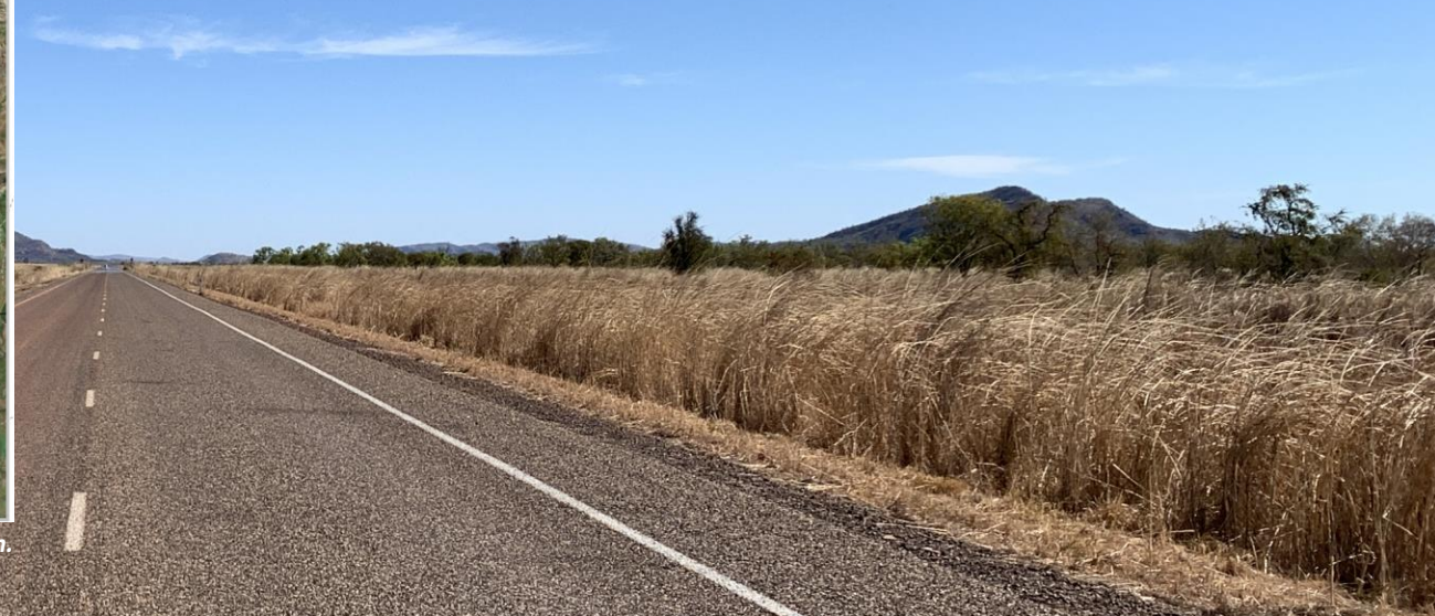
Background: Sealed road connecting the Sorby Hills Project to Wyndham Port.
