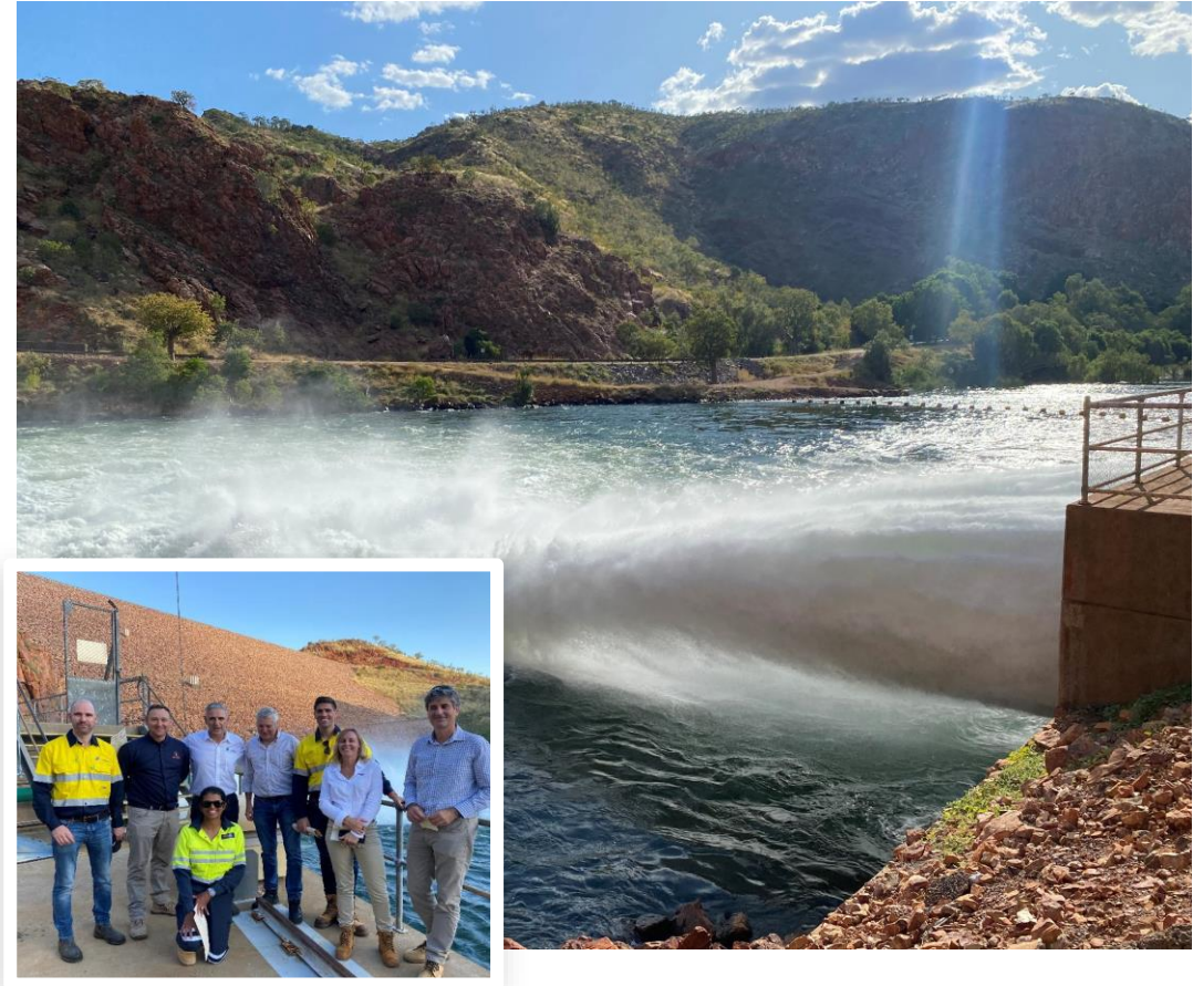
Figure: Members of the Boab and Horizon Power teams on site at the Ord-Hydro Power station.
