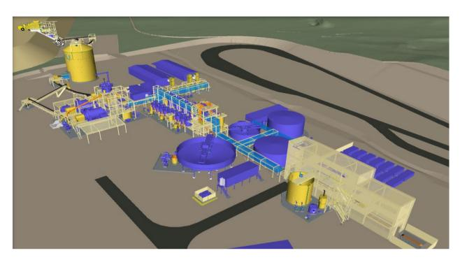
Figure 5: 3D Model of the Sorby Hills Process Plant layout looking northward from the ROM Pad toward the processing facilities and administration buildings.
