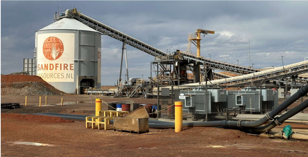
Figure 1: The DeGrussa Processing Plant.
