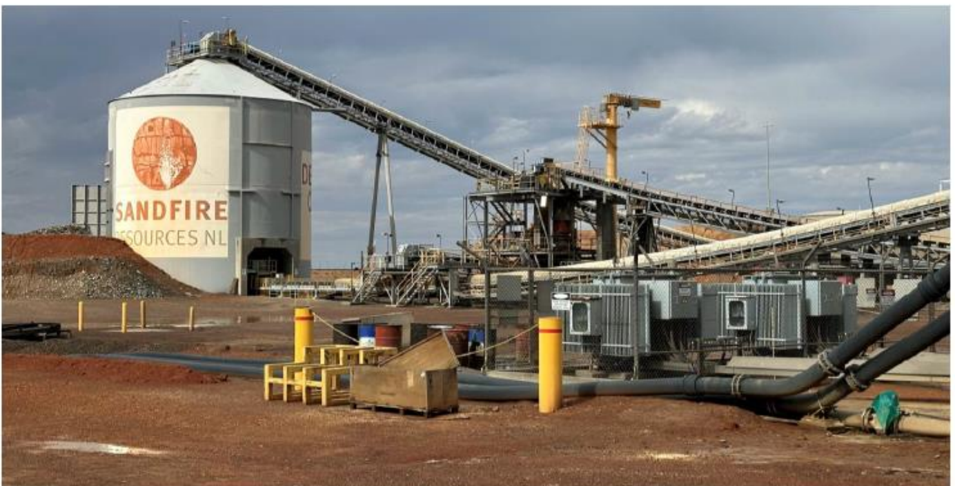
Figure 2: Image of the DeGrussa Processing Plant
