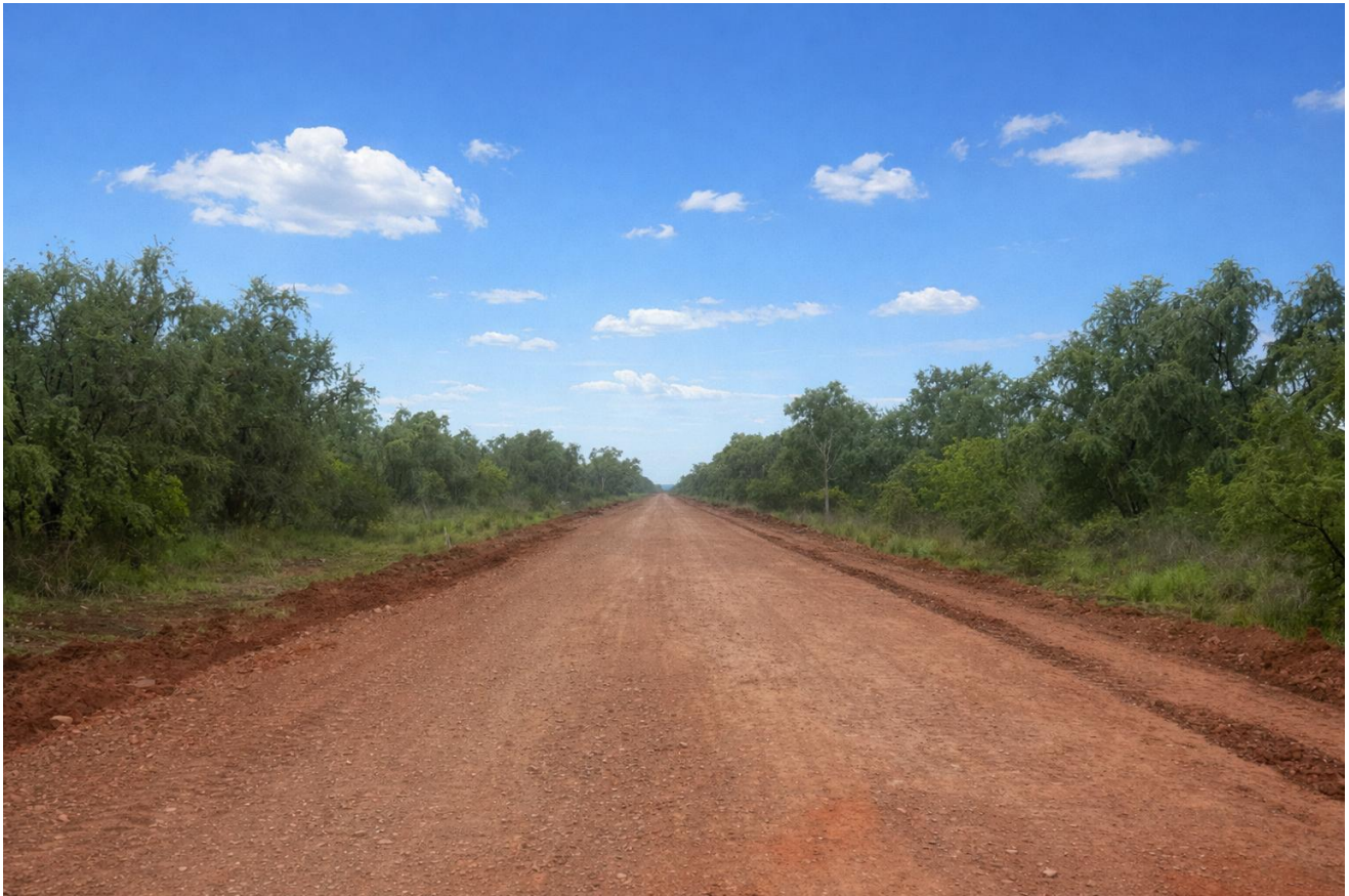
Figure 1: Camp access road sub-base.
